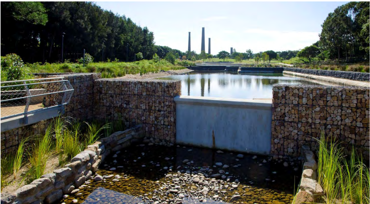
Image: Sydney Park water reuse scheme, Sydney Park, St Peters
