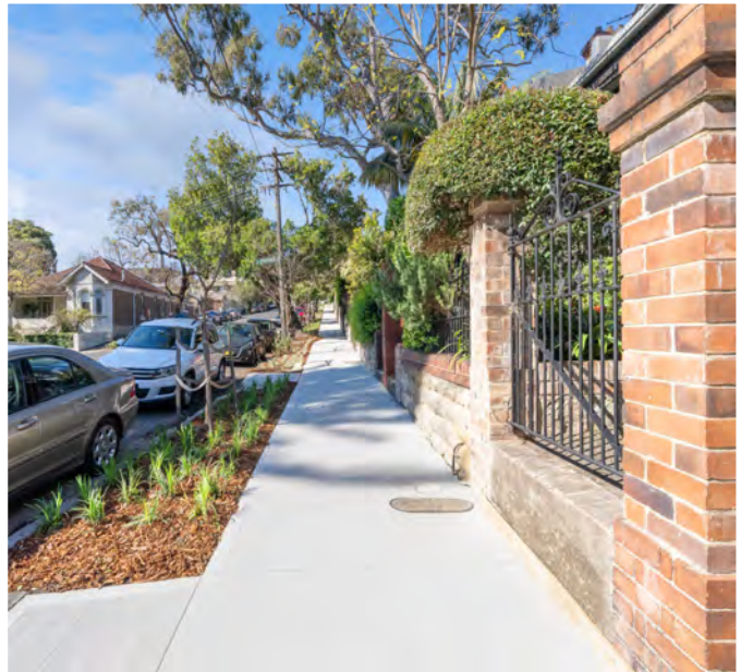
Images: Eglinton Road, Glebe Footway Renewal Works 2021
